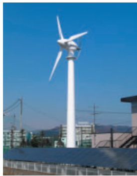
40 kW Wind Turbine Generator System (Installed at the Ashikaga Institute of Technology)
