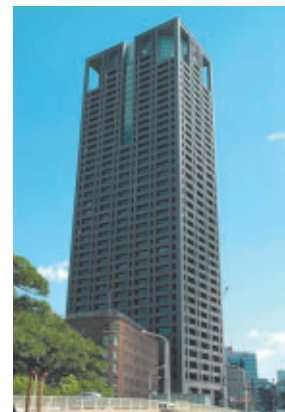
Head Office Building of the Kansai Electric Power Company Number of floors to be processed: From the second floor in the basement to fortieth floor
