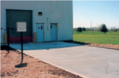
The concrete cover installed in front of the paint solvent recovery facility
