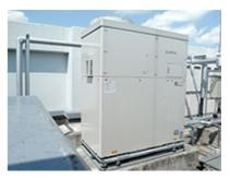
Cogeneration system installed in the Subaru Training Facility
