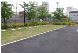
Car park with a flood prevention measure (Gunma Plant)
