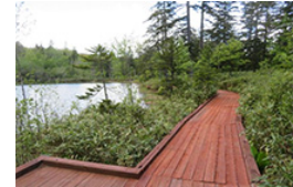
Repaired walking paths around the Matsuyama Marsh
