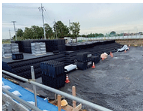
Construction of the storm water detention tank
