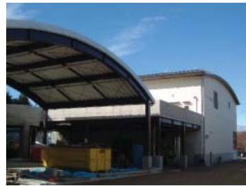
Transit facility (Nasu Town, Tochigi Prefecture)
